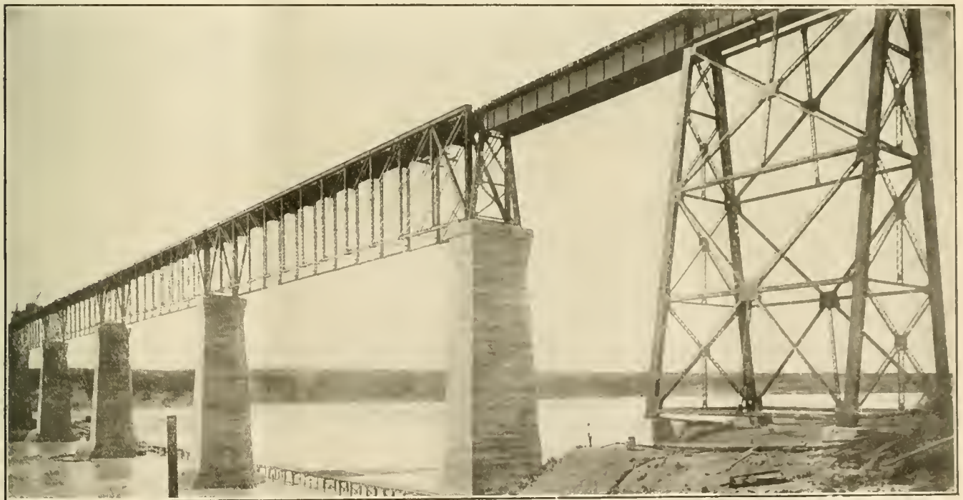
VIEW OF THE RIVER SECTION OF THE OUTLOOK BRIDGE AT LETHBRIDGE. AT THE RIGHT IS ONE OF THE NINE LAND TOWERS.
